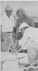
INSTRUCTOR F. Geerman sets block in place.
